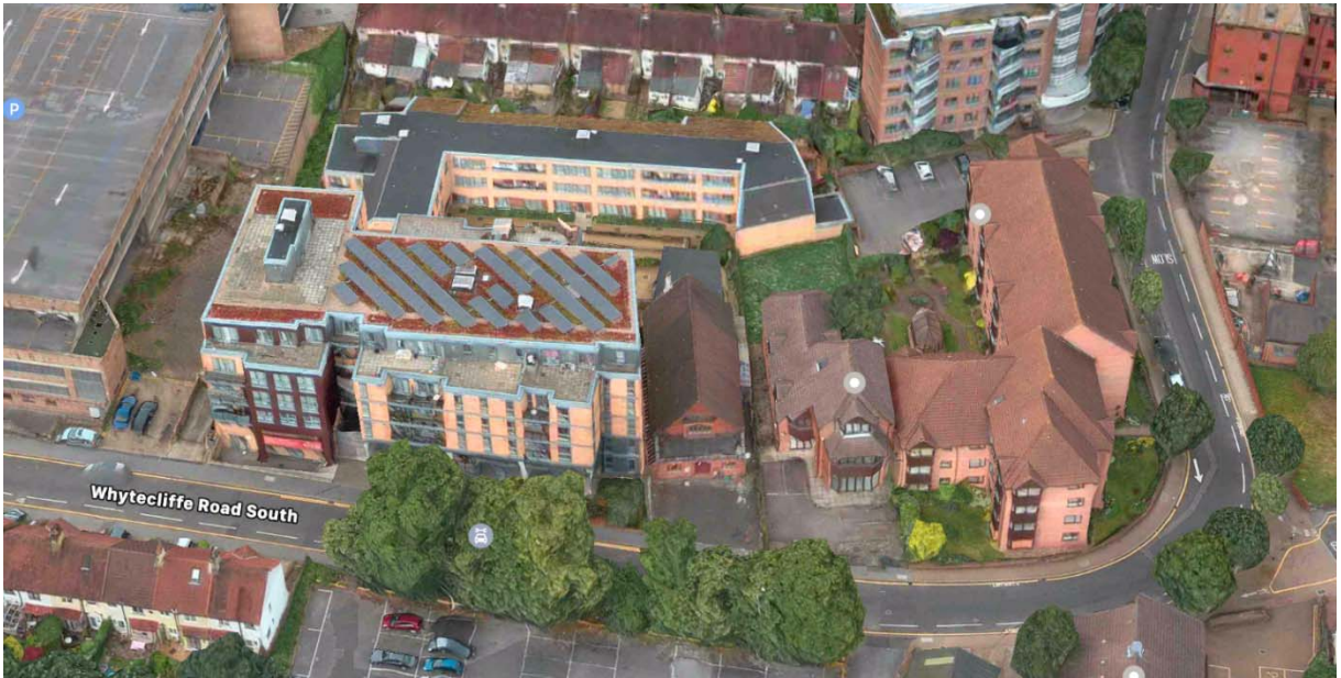
Figures 2 and 3: Images of existing buildings surrounding the site.
