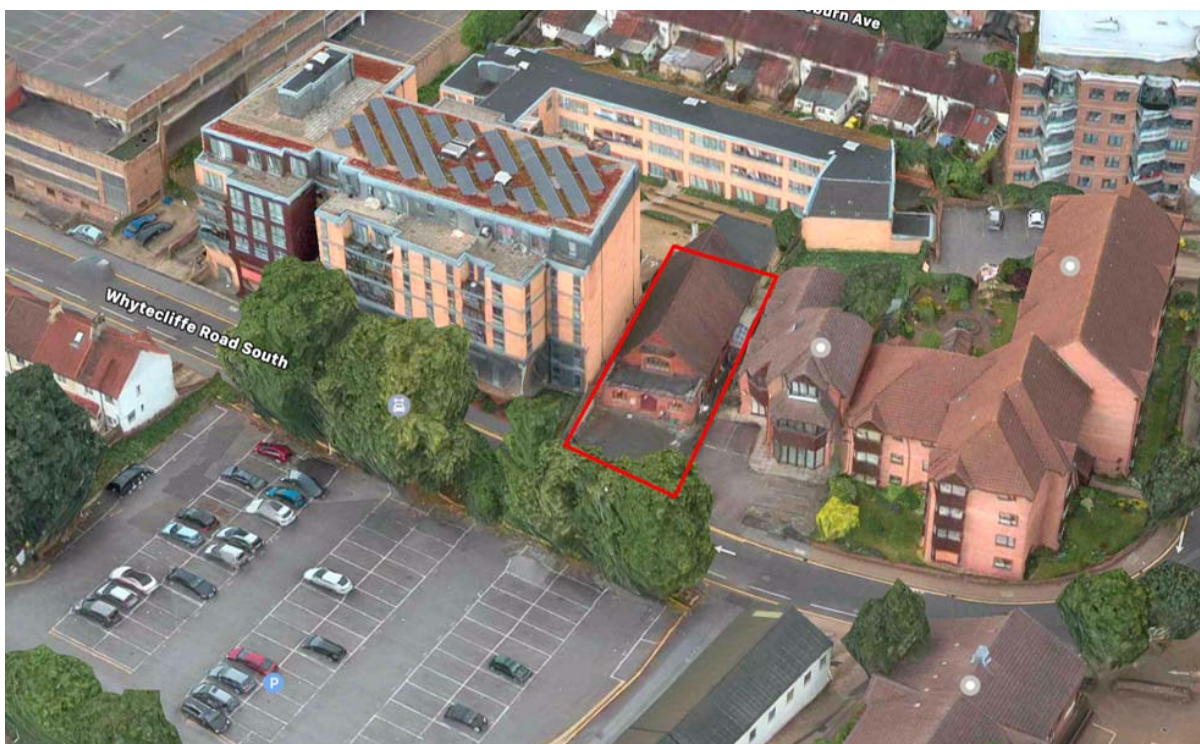
Figure 1: Aerial street view highlighting the proposed site within the surrounding street-scene
